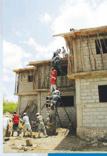
The concrete bucket brigade goes up a ladder as a new building is constructed in Jamaica
