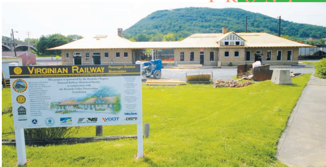
The Virginian Station station under renovation
