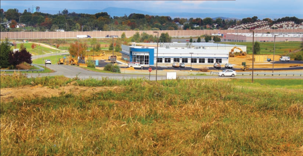
Aeroprobe's new facility under construction in Christiansburg.
