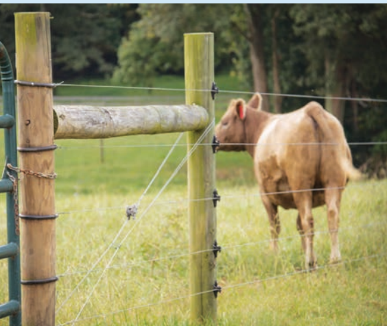
Installing livestock fencing along waterways creates a long-term improvement to the farm's infrastructure.
