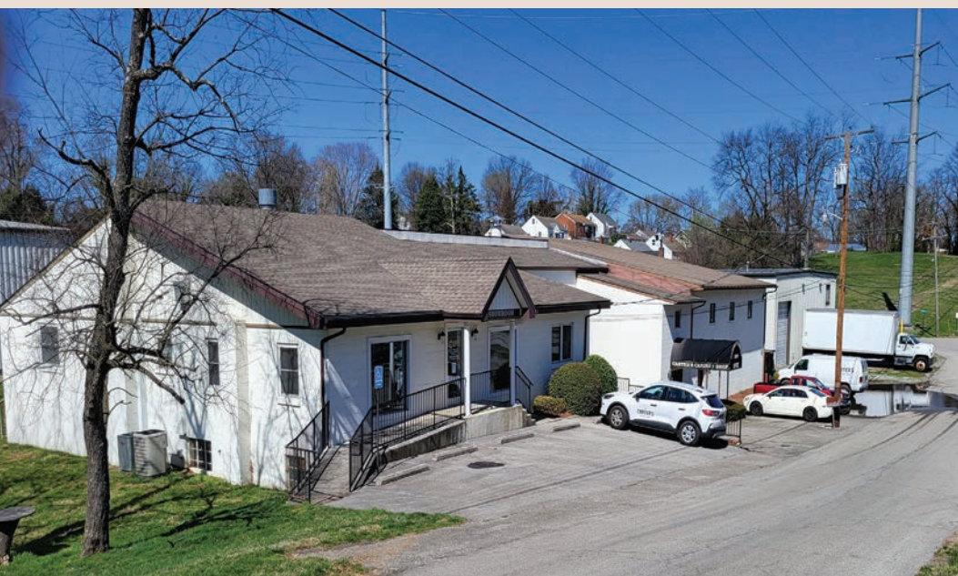
Carter's Cabinet Shop has grown from the basement of a mid-sized Roanoke home to a 12,000-square-foot business. The original home business is to the left.
