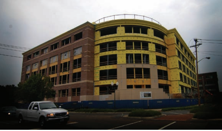
A Carilion Clinic building under construction
