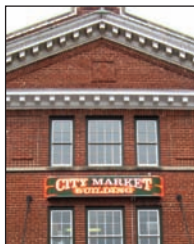
City Market Building
