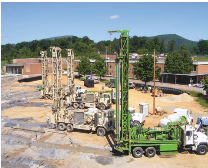
Richard Simmons workers put in the geothermal grid at Northside High
