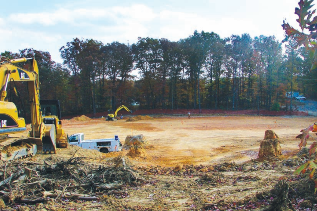
Warm Hearth Village Center under construction.
