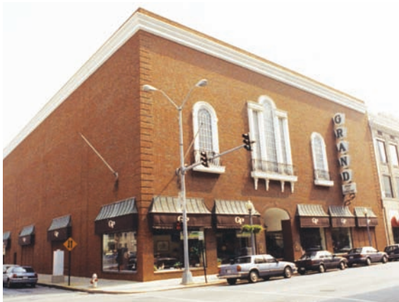
The Hancock Building—which was recently returned to its 1920s façade—was home for Grand for many years in downtown Roanoke.
