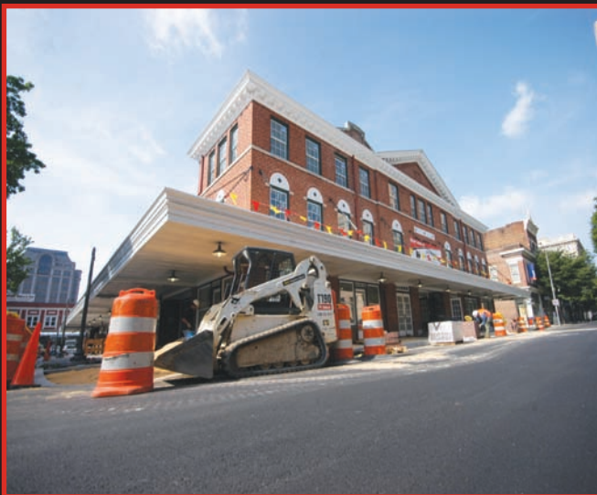
Downtown access restricted from construction
