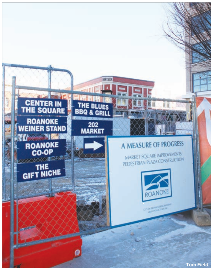
Market Square renovation
