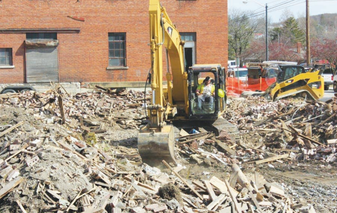
Construction begins at Jackson Park Inn and Conference Center in Pulaski
