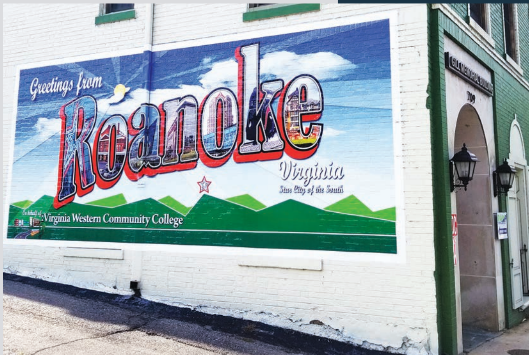
Iconic graphic adorns renovated Gill Memorial Building at 709 Jefferson Street in Roanoke, home to the RAMP suite and RBTC (Roanoke) office.
