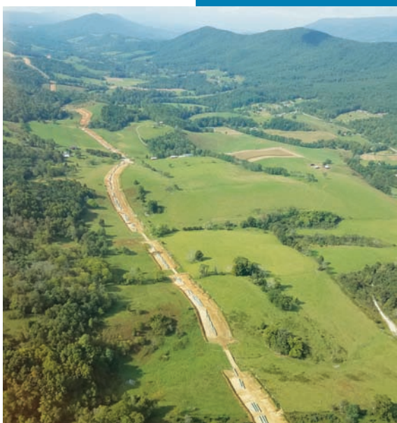
42-inch diameter pipe sections in place
