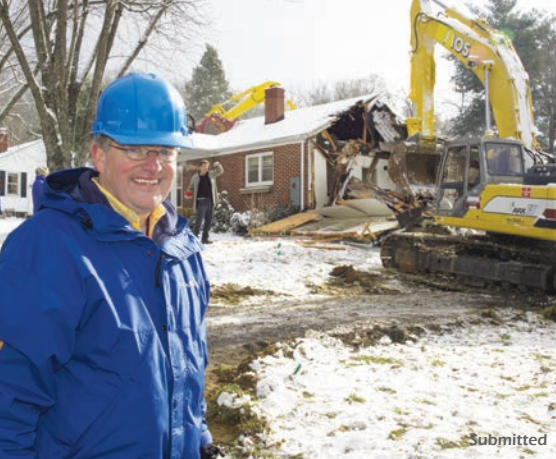
The ABC home build was done in freezing temperatures and snow/ice.
