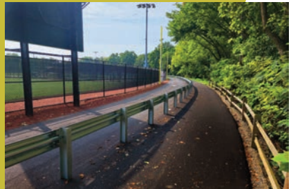
Salem Street Department helped with the perimeter rail installation.
